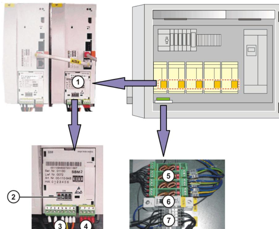
Fig. 3-3: Example: SBM2 components in the top-mounted cabinet
